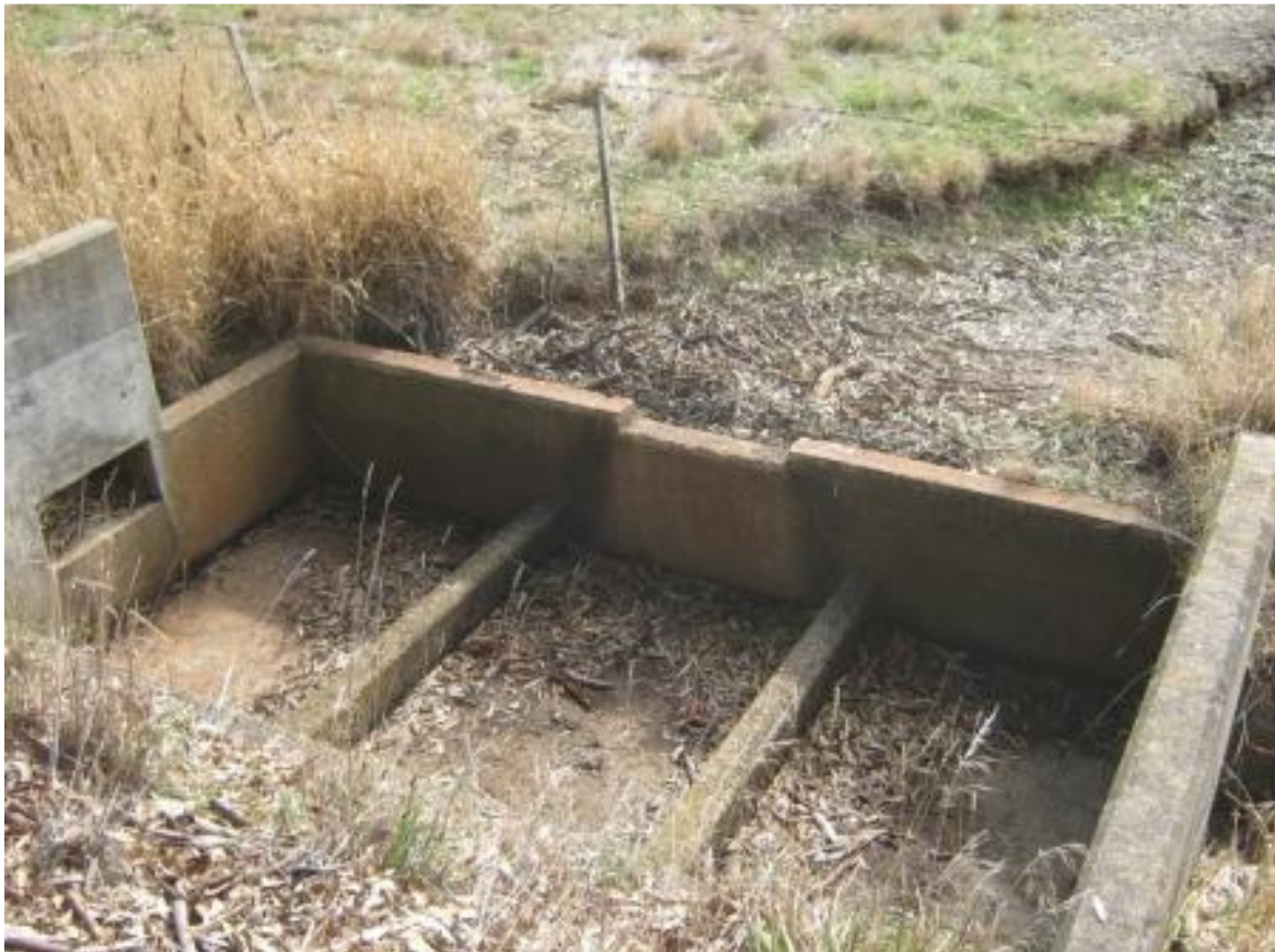
Figure 11 - Broad Crested Weir at U/S of Road
